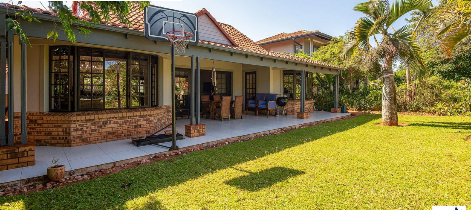
3 Bedroom Self Catering House, Zimbali Coastal Resort, Forest Estate Villas
